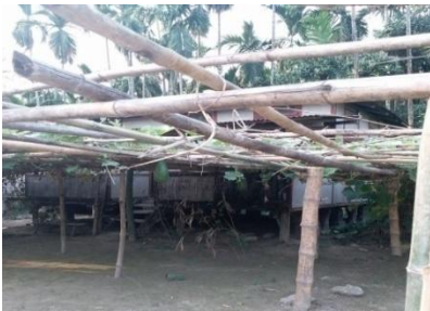
186. Chang bangle (raised platform) and janla (post and fencing of bamboo poles)
