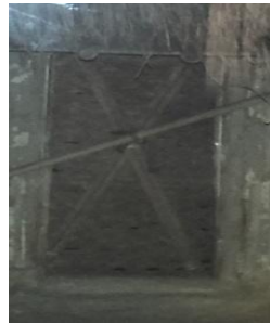
187. Door made of woven bamboo mat and lock made of oua (bamboo pole) called ' pala thokon '
