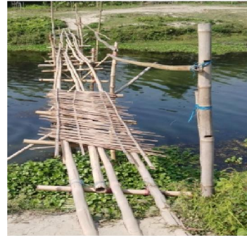
193. Traditional bridge made of woven bamboo sticks and poles.
