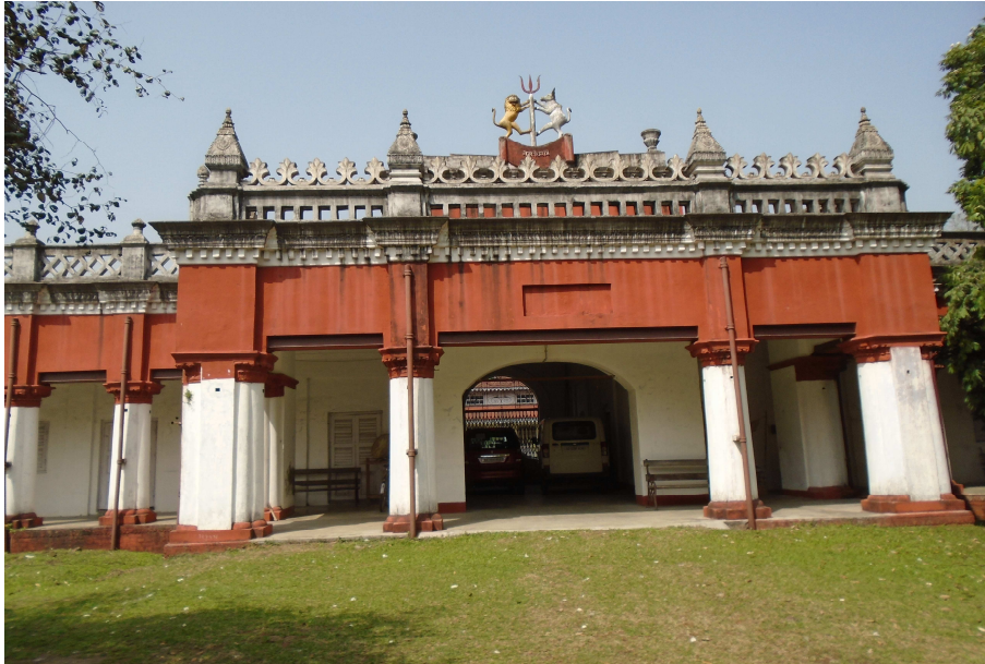
Main entrance of Bijni Raj Palace
